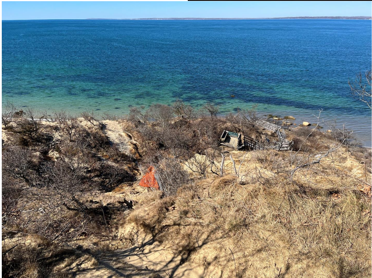
Photograph 1. Slumping of the coastal bank at the site has compromised the wooden stairway system to access the beach.
