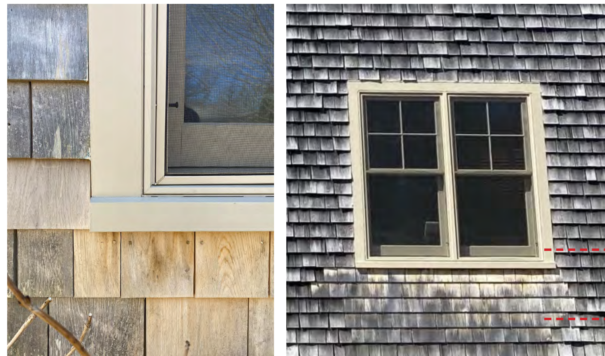
NEW WINDOWS TO MATCH STYLE AND COLOR OF EXISTING WINDOWS. CEDAR EXTERIOR SHINGLES TO MATCH EXISTING.
