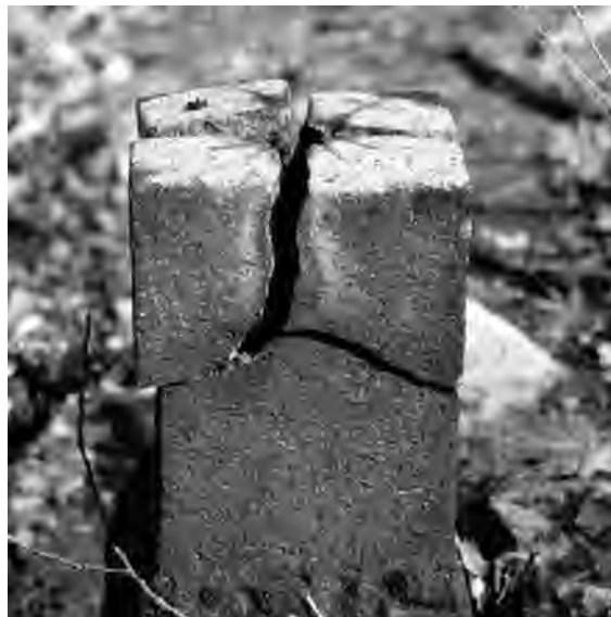
Rust jacking at former fence post support, East Parish Burial Ground, Newton [left] Chocksett Cemetery, Sterling [right]
