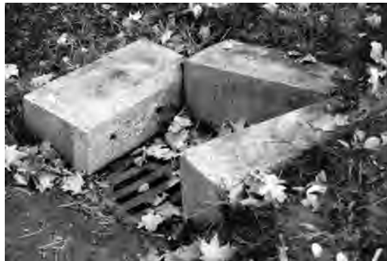
Marker bases used as drain edging, Cambridge Cemetery, Cambridge
