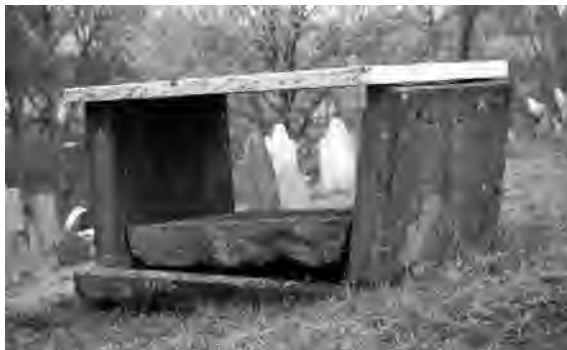
Damaged box tomb, Old Hill Cemetery, Newburyport
