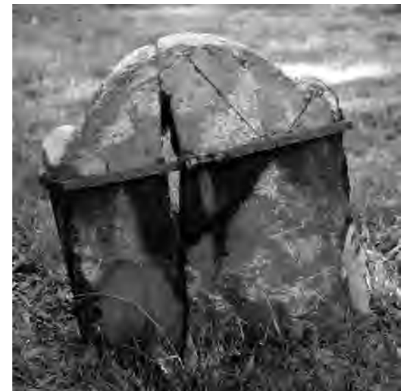
Iron strap repair, Spring Hill Cemetery, Marlborough
