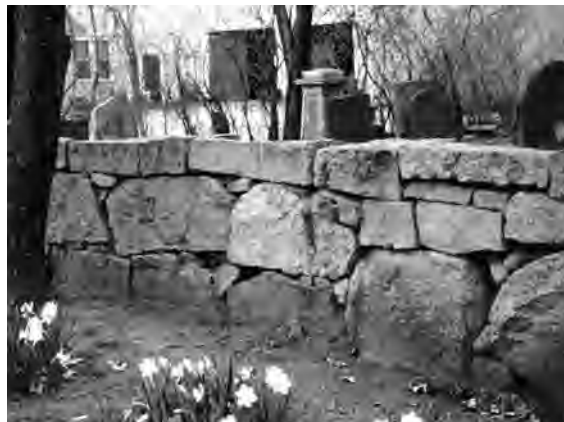
Dry laid stone wall, Old Burying Grounds, Littleton
