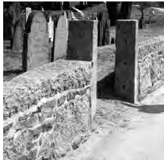
Mortared stone wall, Old Burial Ground, East Bridgewater
