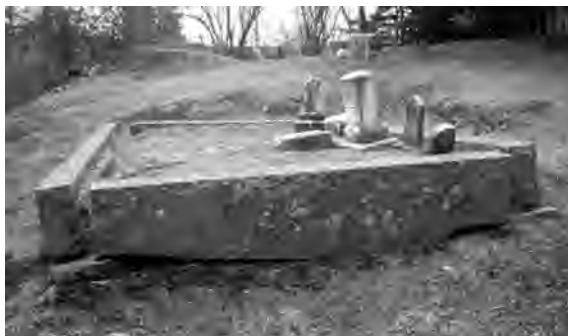
Settlement and overturning at family plot edging, Old Burying Grounds, Littleton
