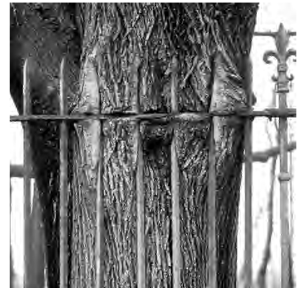
Tree growth at iron fence, Glenwood Cemetery, Everett
