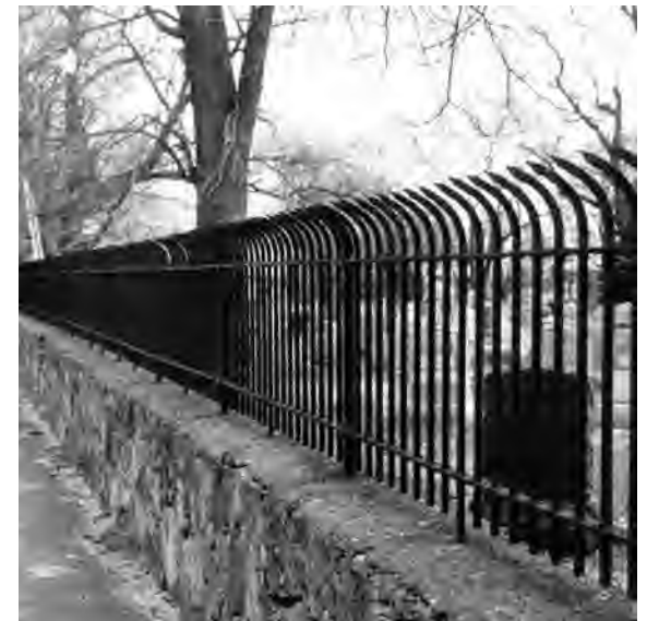
Iron fence on stone masonry wall, Glenwood Cemetery, Everett
