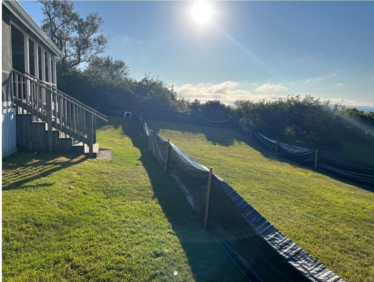
Demolition of the entire house. New house is outside jurisdiction
