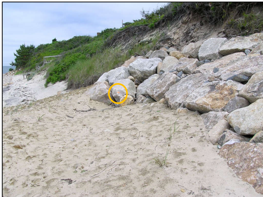
Monitoring Station #1: Beach at elevation 8.0 ft NGVD (1 ft below survey mark) on June 24, 2009.
