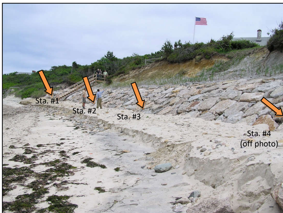
Overview of revetment and initial beach nourishment June 24, 2009; view looking northeast.
