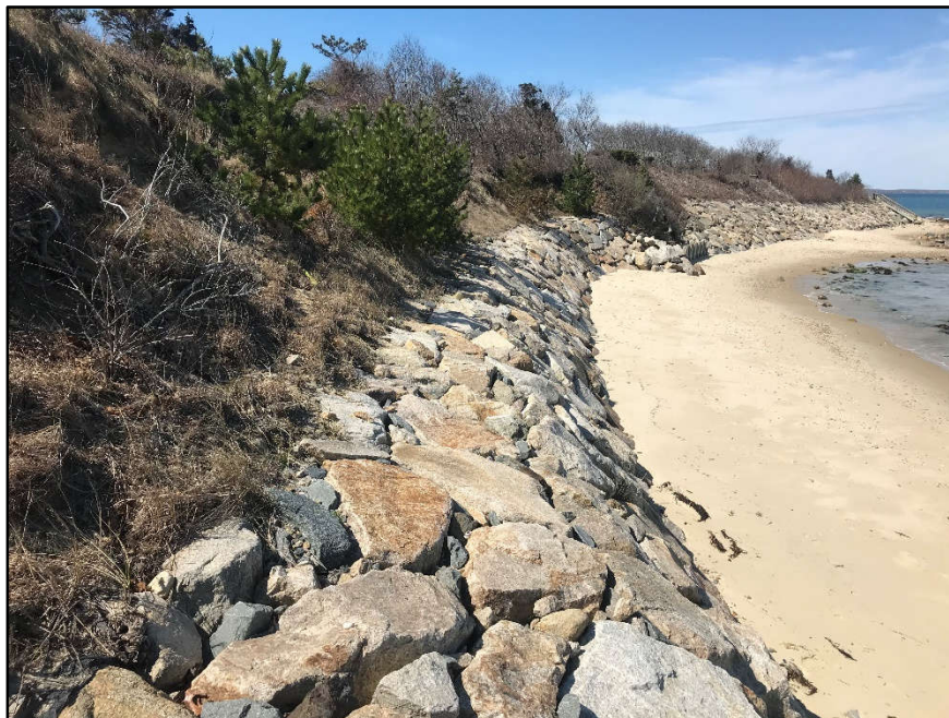
Overview of revetment and coastal beach on April 14, 2020. View looking southwest.
