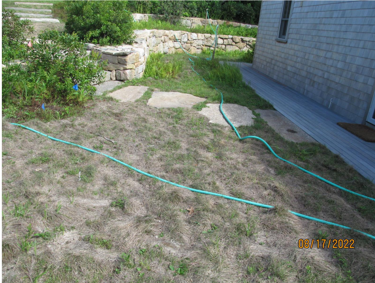
new stone stairs and retaining wall. ( bad picture. sorry)
