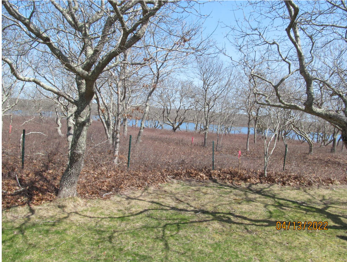
staking for new house
