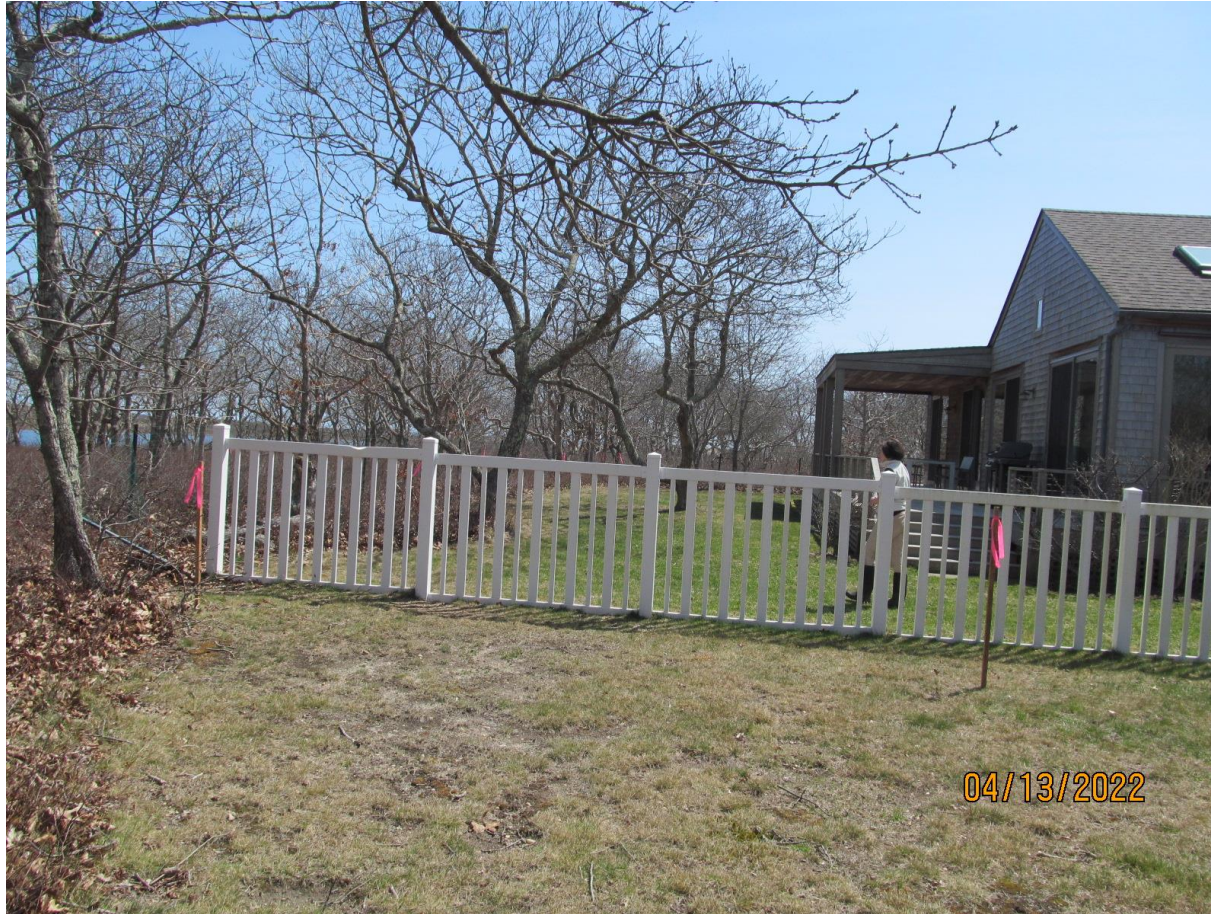
staking for new house
