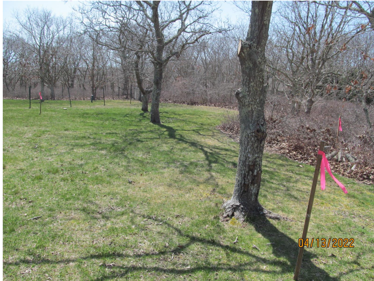
Staking for garage
