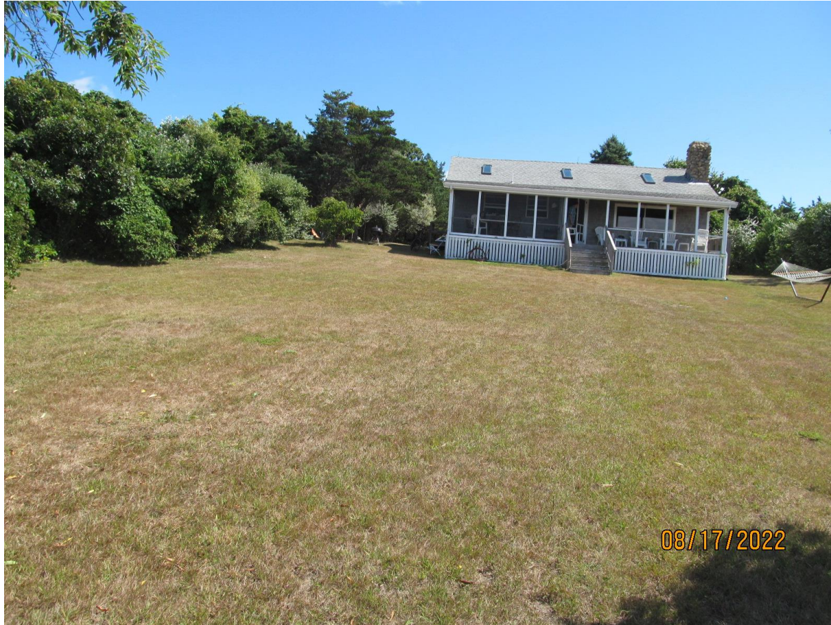
view from stairs at top of bank back to the house. Addition is outside the buffer zone to top of the coastal bank.
