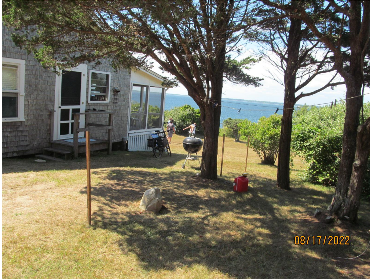
Stakes represent location of dining room and deck addition
