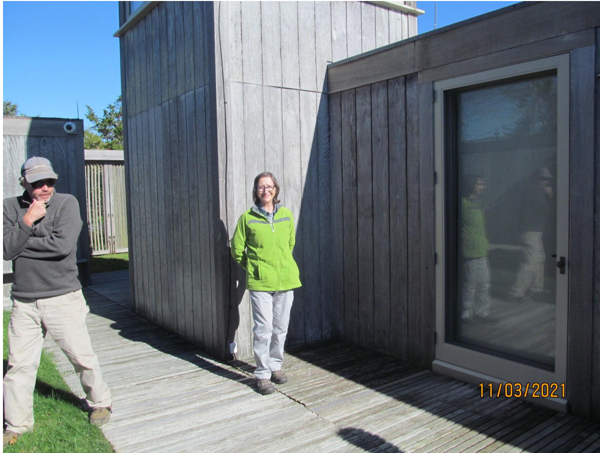
Building 3. Kitchen. Donna is standing in the 20 sq. ft addition for powder room
