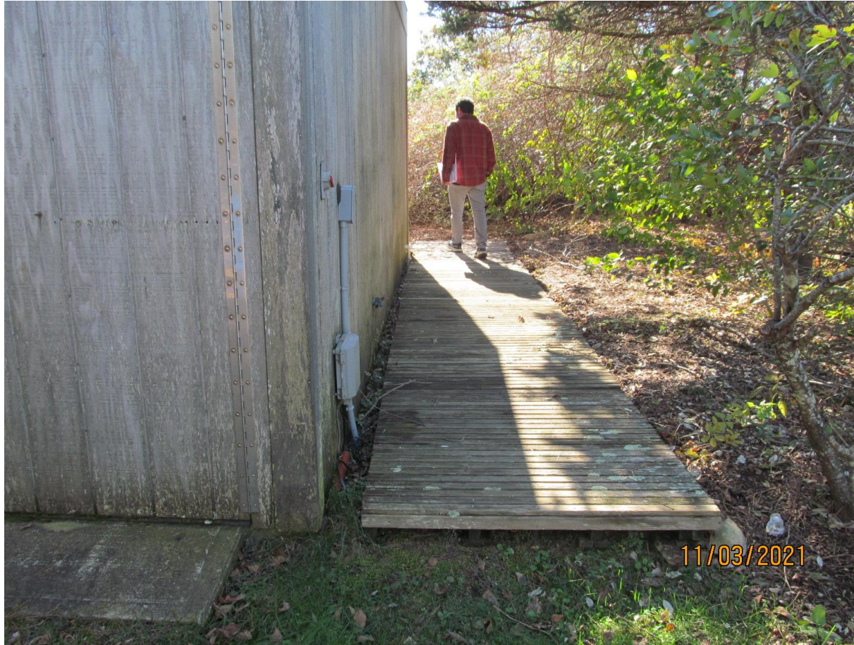
Boardwalk around compound
