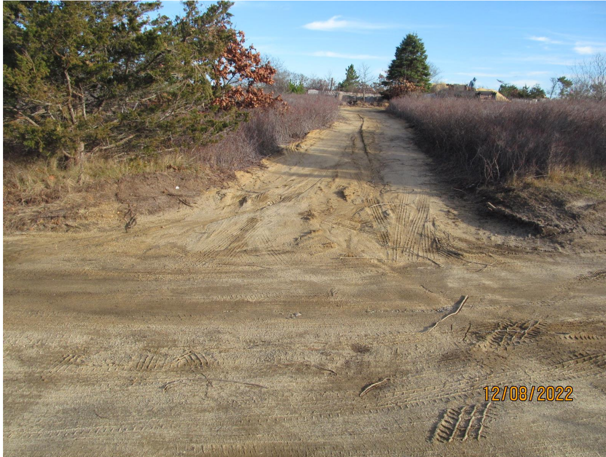
New driveway at 216 MPR. May be contributing to surface runoff at 208 MPR
