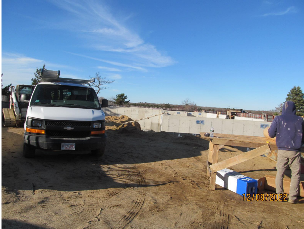
new house construction
