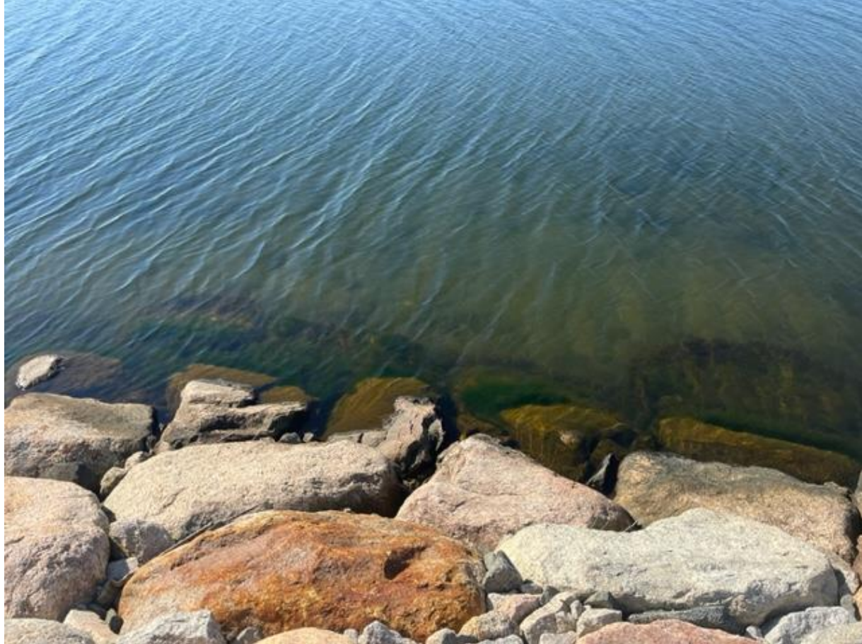
two rows of toe stones under water. pond is closed
