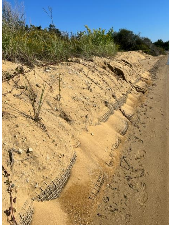
Revetment north side
