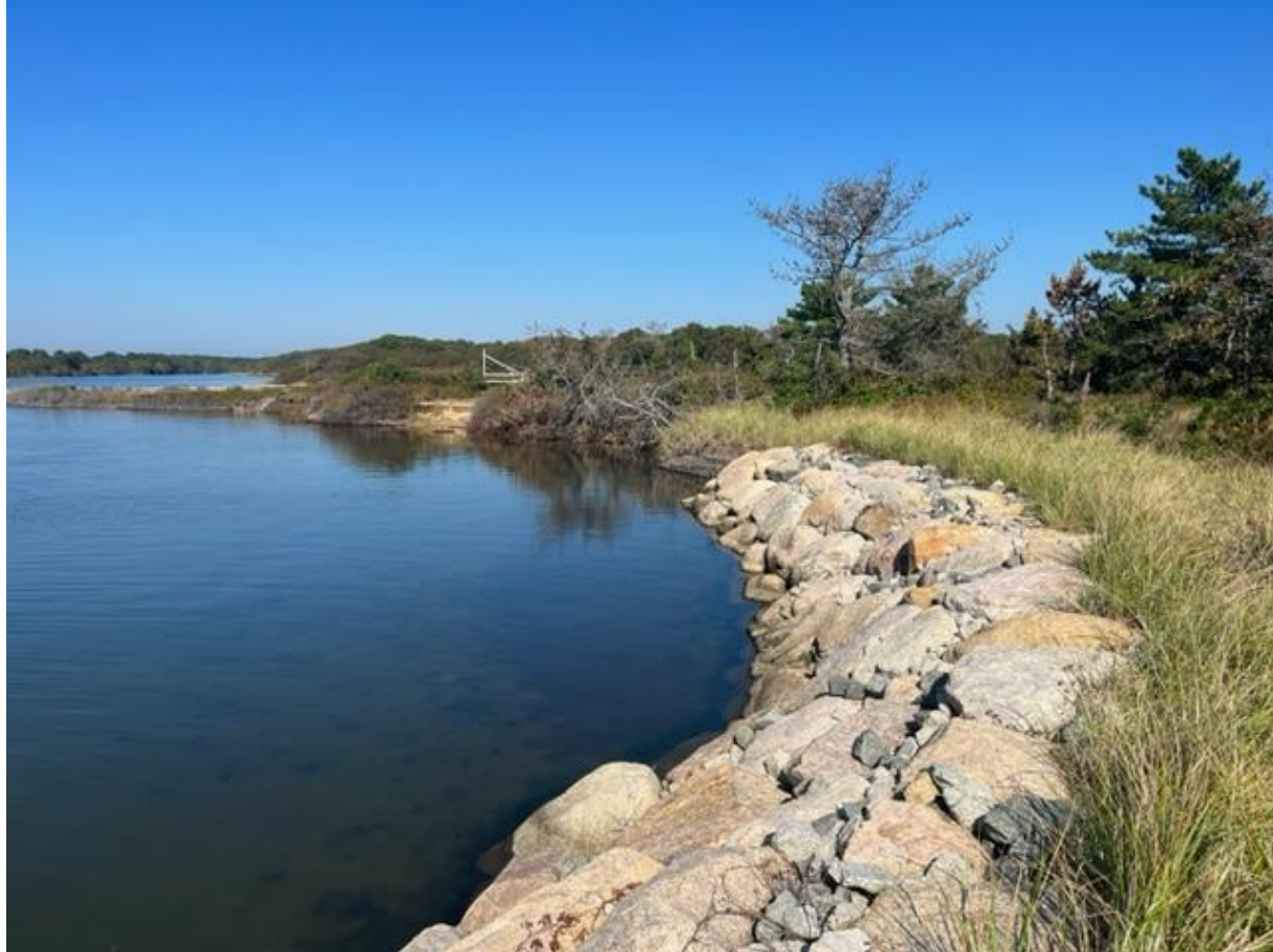
North end of revetment
