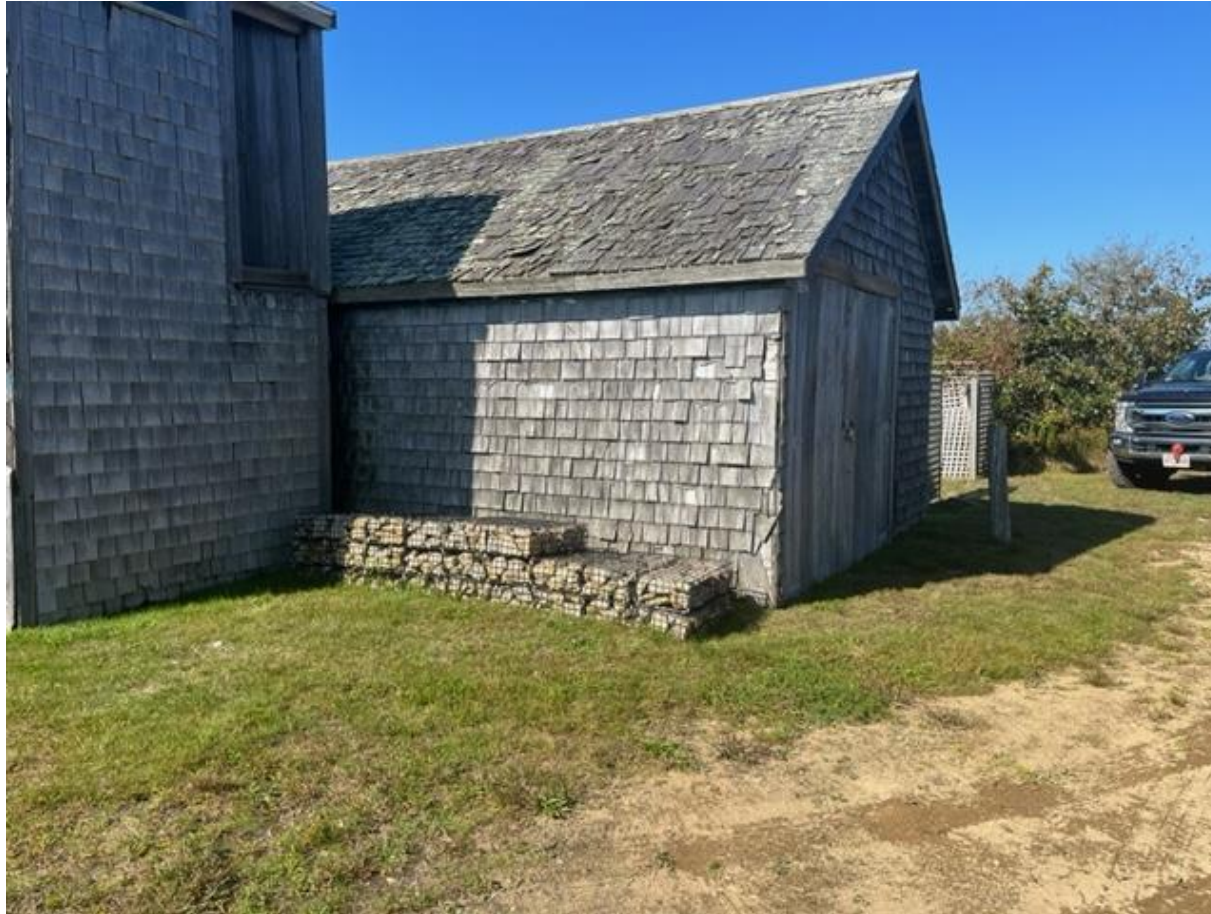
New gabions resting against the house
