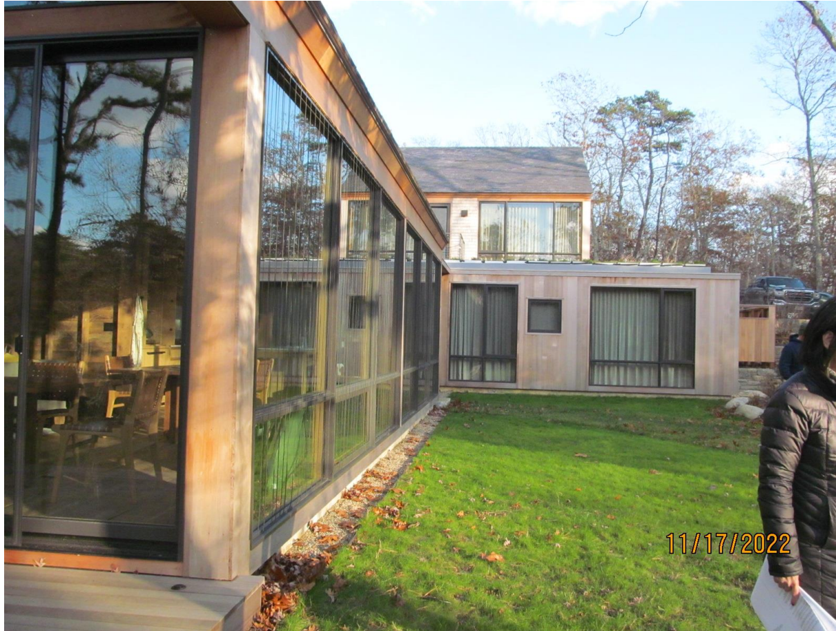
Drip line for roof runoff
