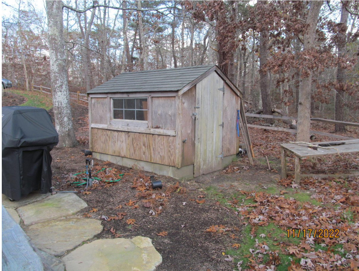
Well house wasn't moved to much work to rebuild foundation to move it a foot or two back.
