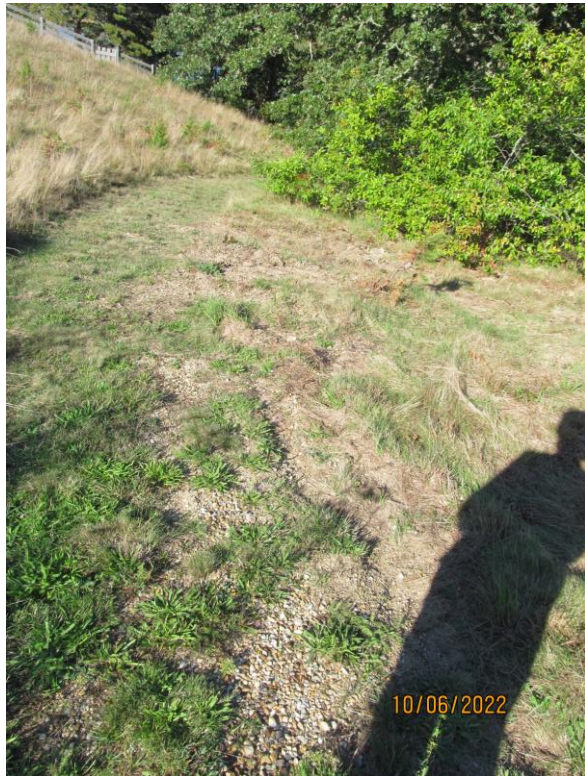
Old path. Area not well vegetated
