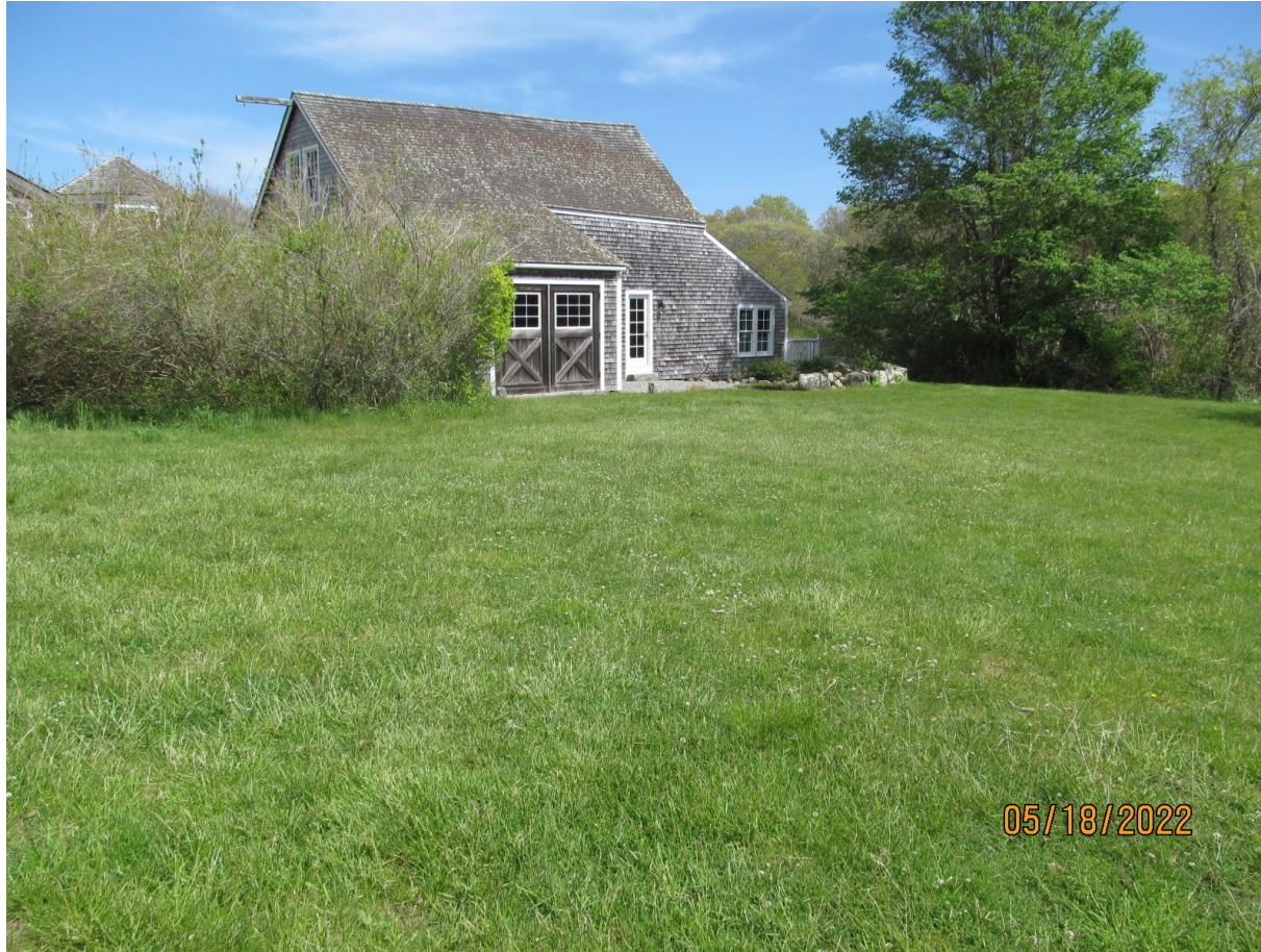
side of barn from the driveway Portion of barn was removed
