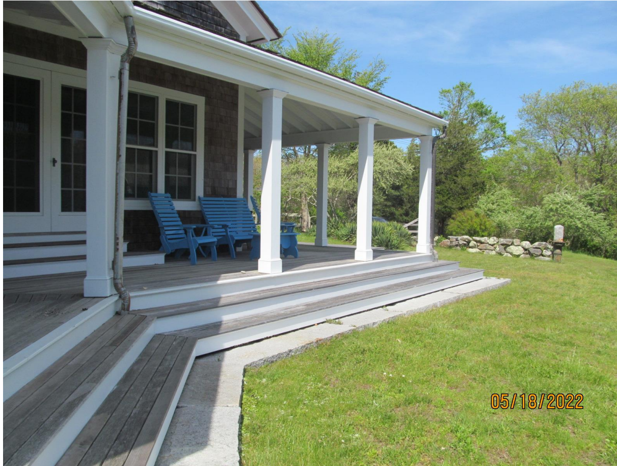
Order required plan to control roof runoff. Gutters installed
