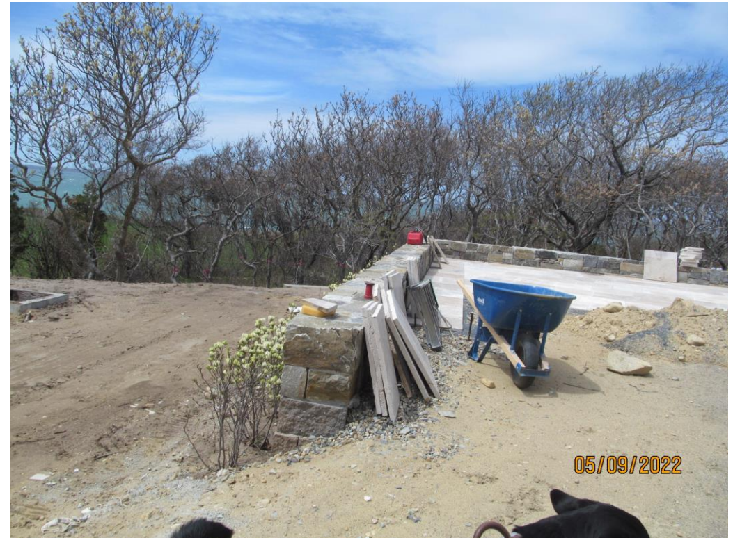
View from west corner of terrace looking east
