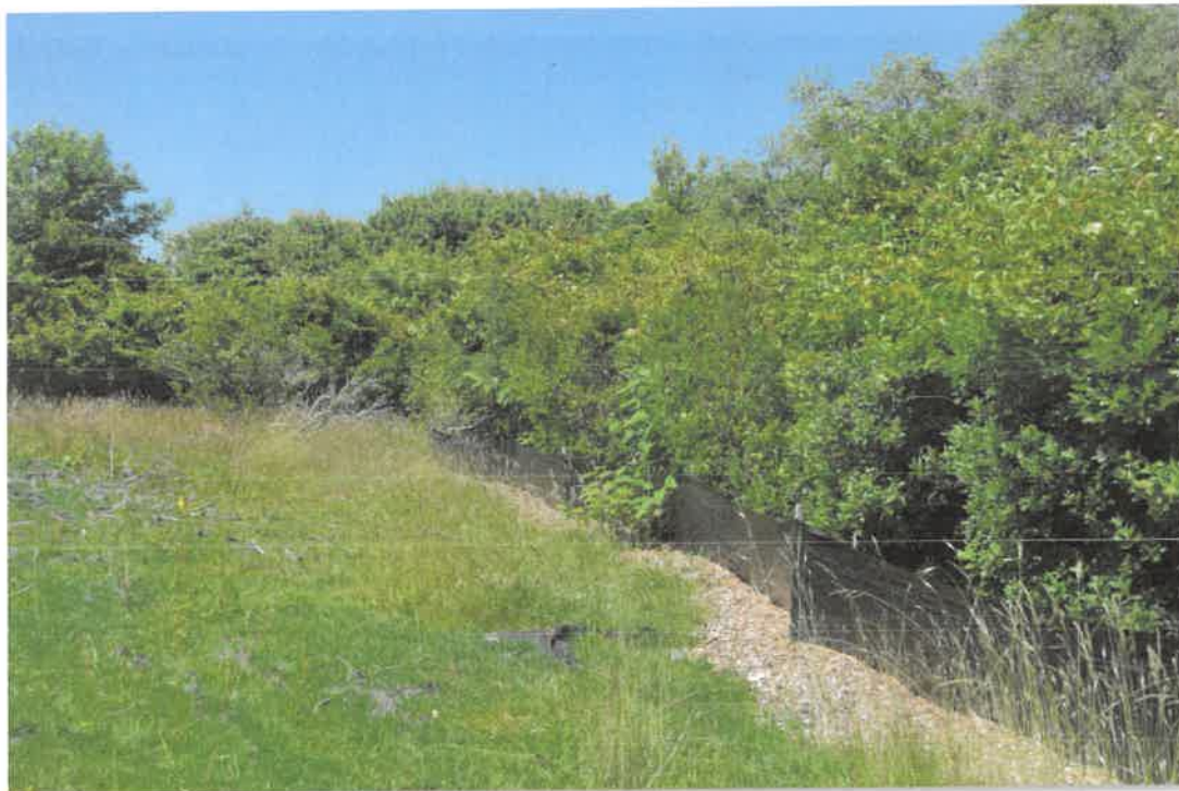
Wetland boundary with erosion control barrier
