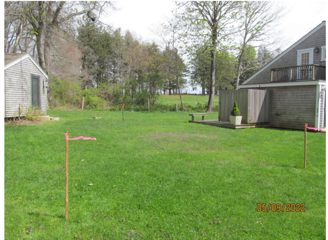
Staking for pool and patio and addition
