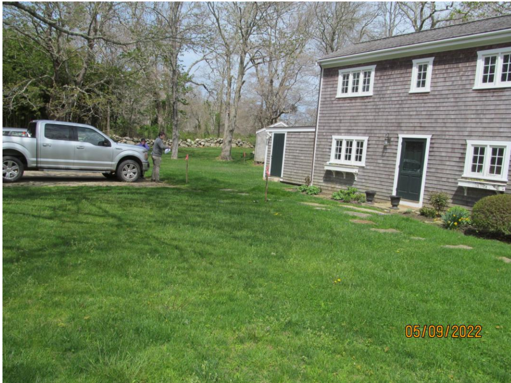
Staking near truck marks front of addition
