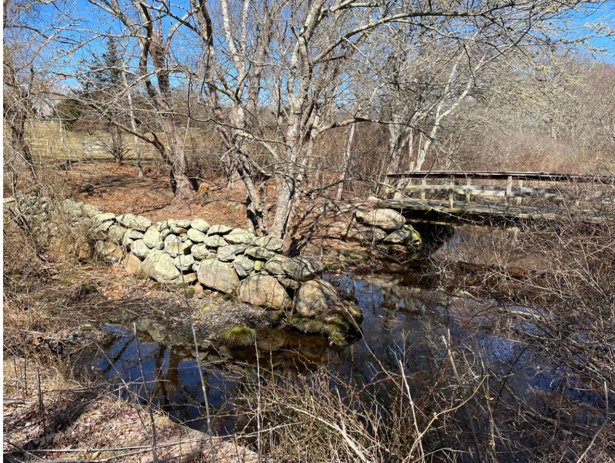
bridge over Tiasquam taken from Murpshy Road. Looking toward Harley property
