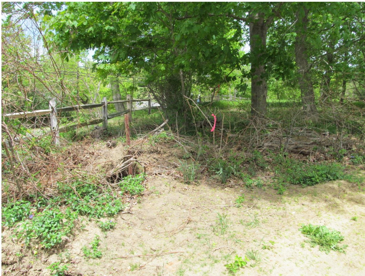
Flagged area to be cleared
