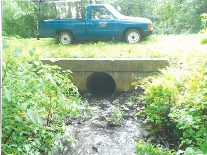
Upstream Face of culvert on Witch Brook at North Road
