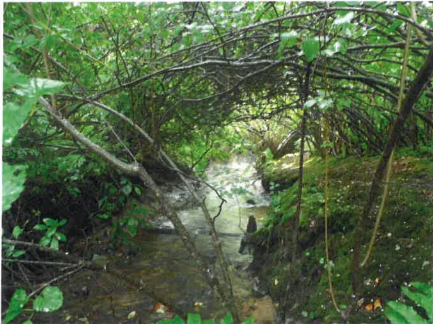
Photo 5: View looking upstream from the culvert on Tiah's Cove Road
