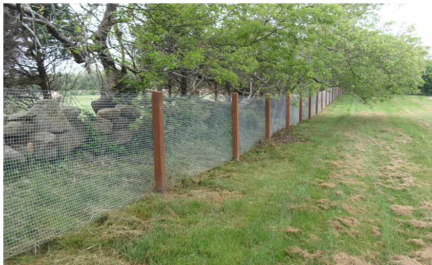
4FT MESH FENCING WITH SERVICE GATE- 1" SQUARE MESH FENCING ON CEDAR POSTS PT POSTS WITH CEDAR TRIM
