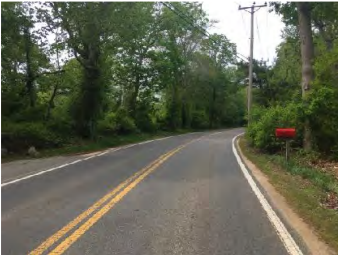
Looking east at entry as you enter
