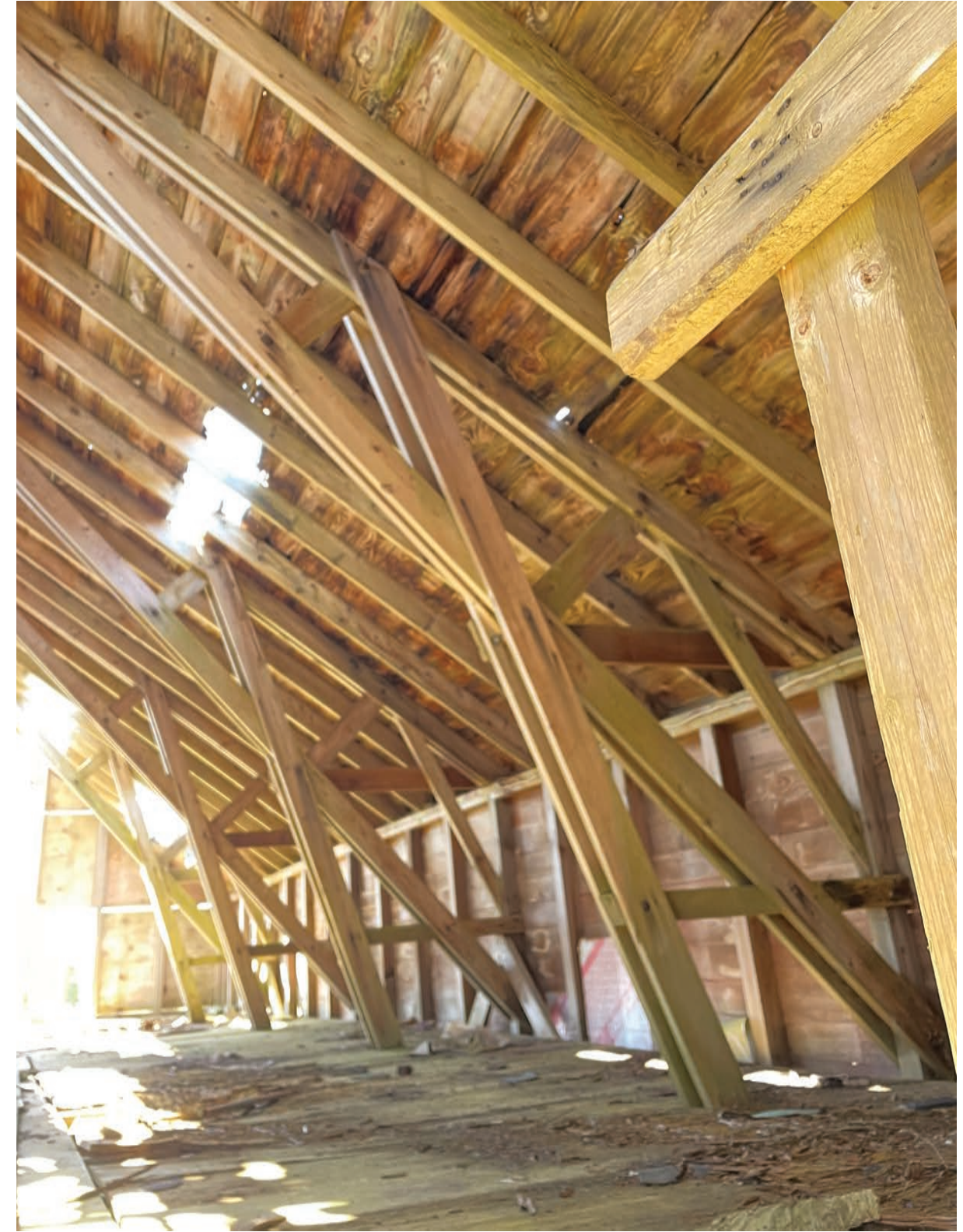
EXISTING BARN TRUSS
