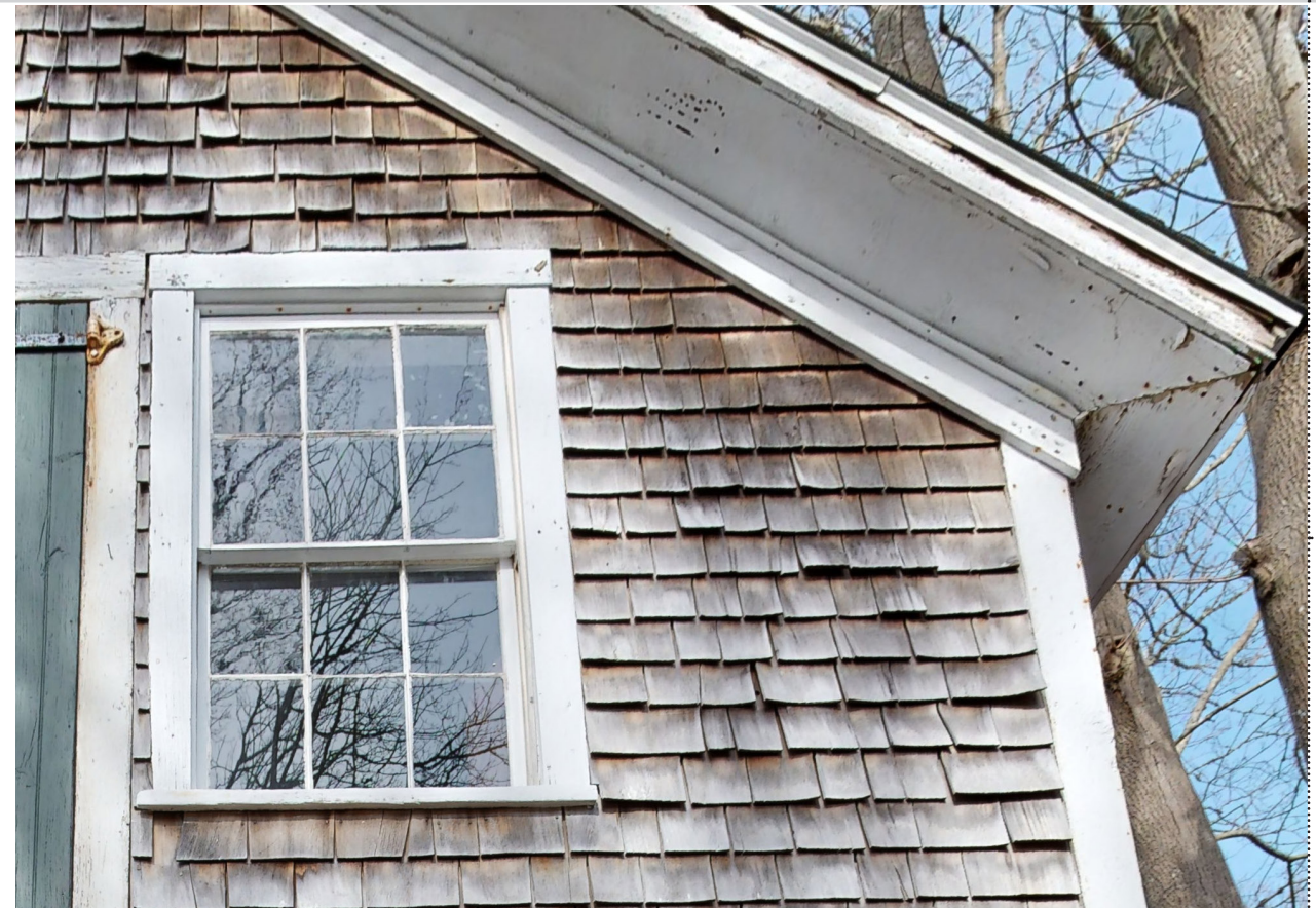
Existing Exterior Trim Details to be Replicated
