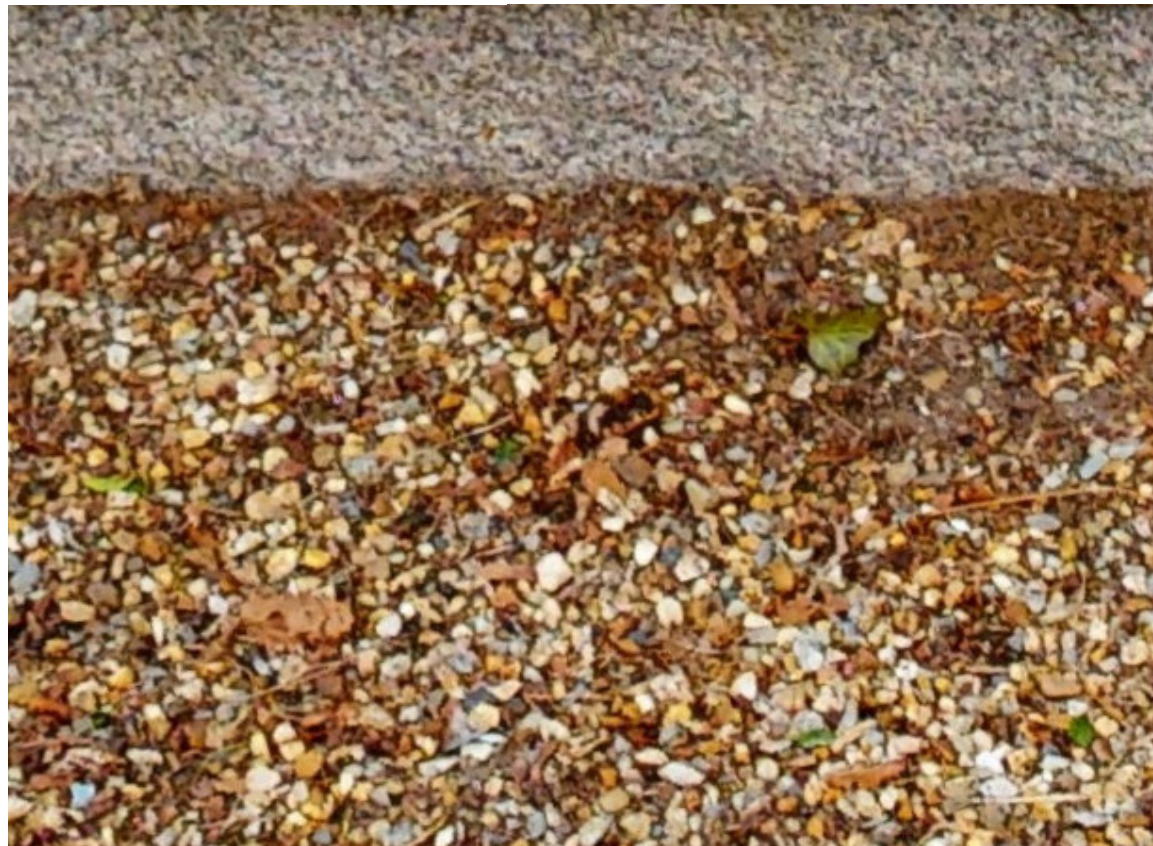
Driveway Material - Granite Apron & Pea Stone
