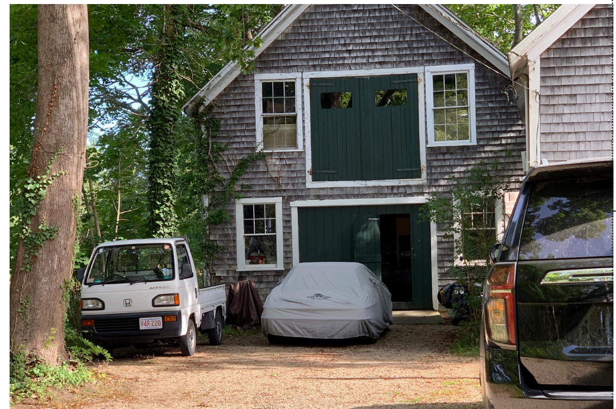
EXISTING BARN & GUEST HOUSE VIEW FROM DRIVEWAY
