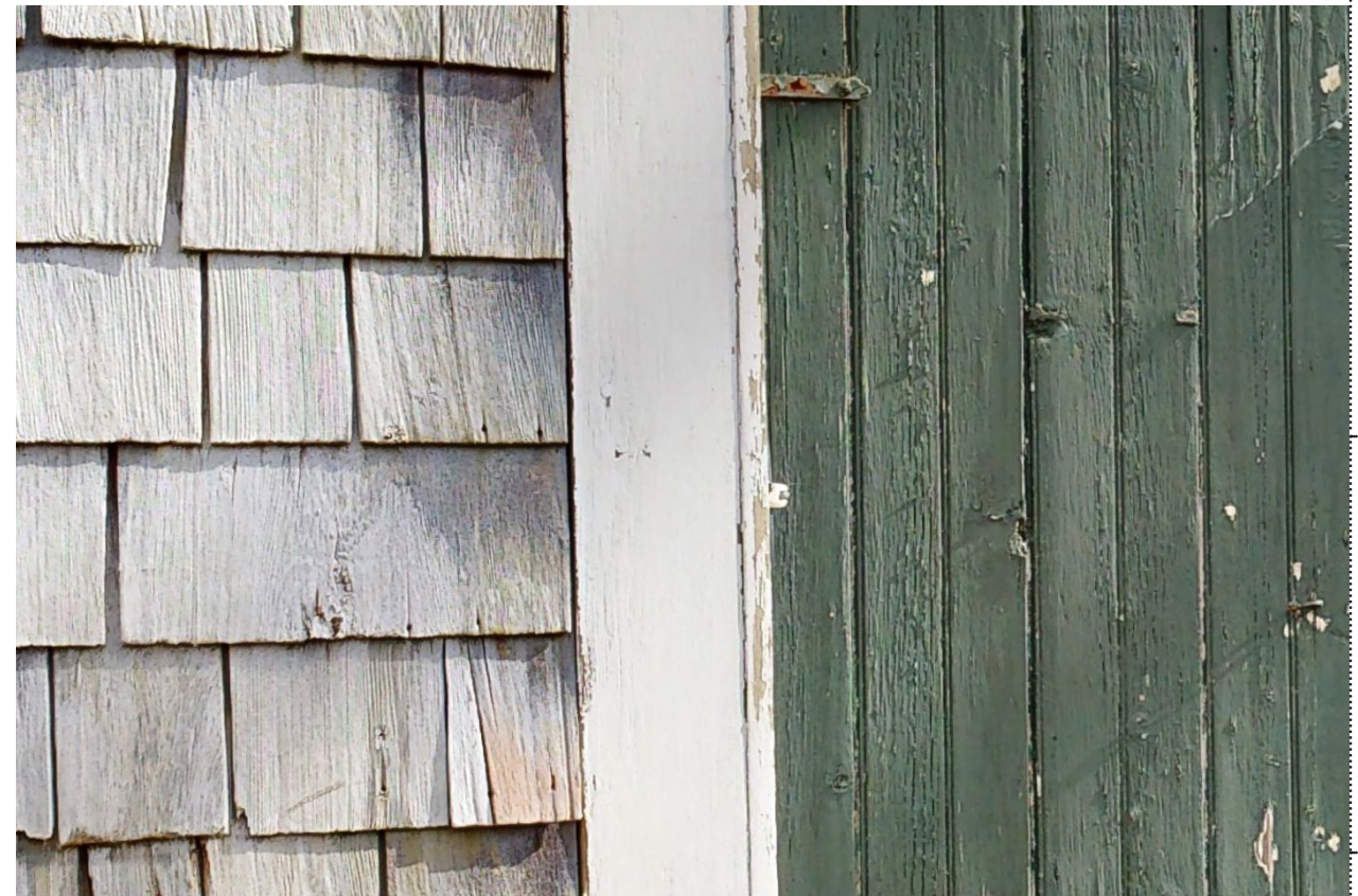
Existing Exterior Siding Materials to be Replicated
