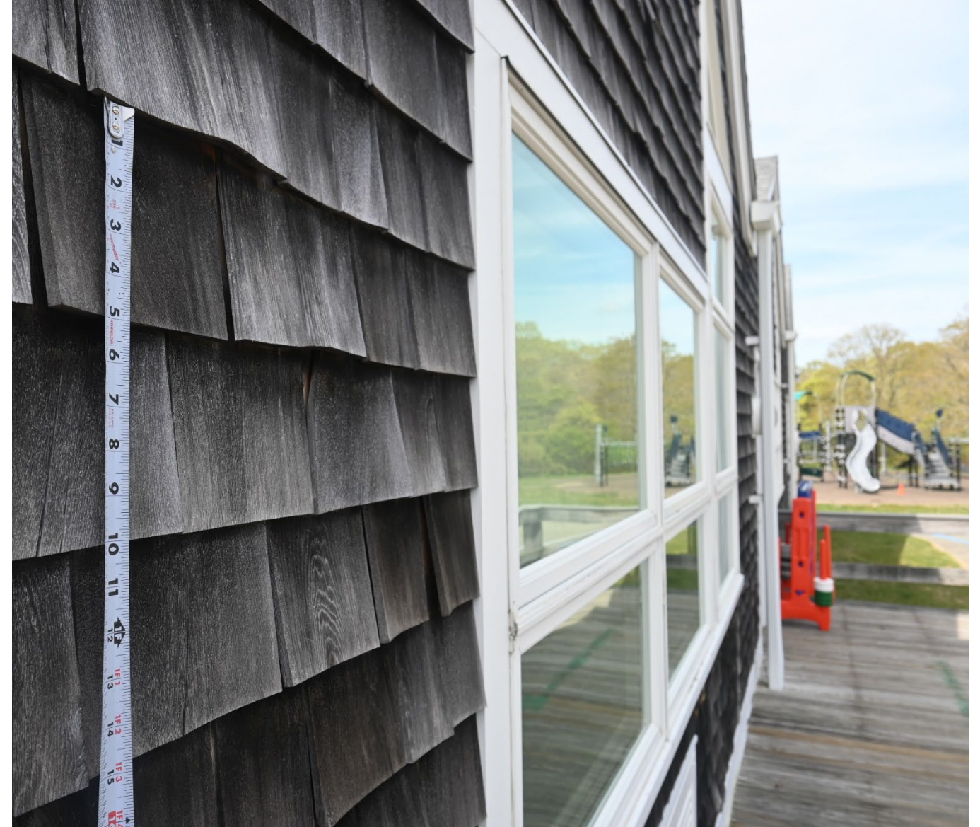
WARPED AND WEATHERED CEDAR SHINGLES NEARING THE END OF THEIR LIFE.
