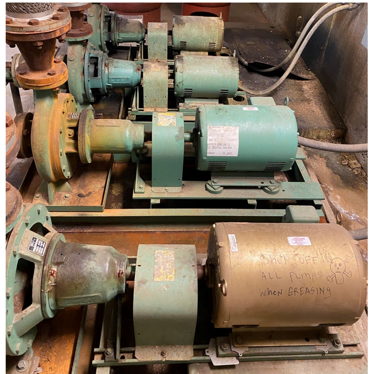
FOUR EXISTING PUMPS, TWO NOT WORKING.
