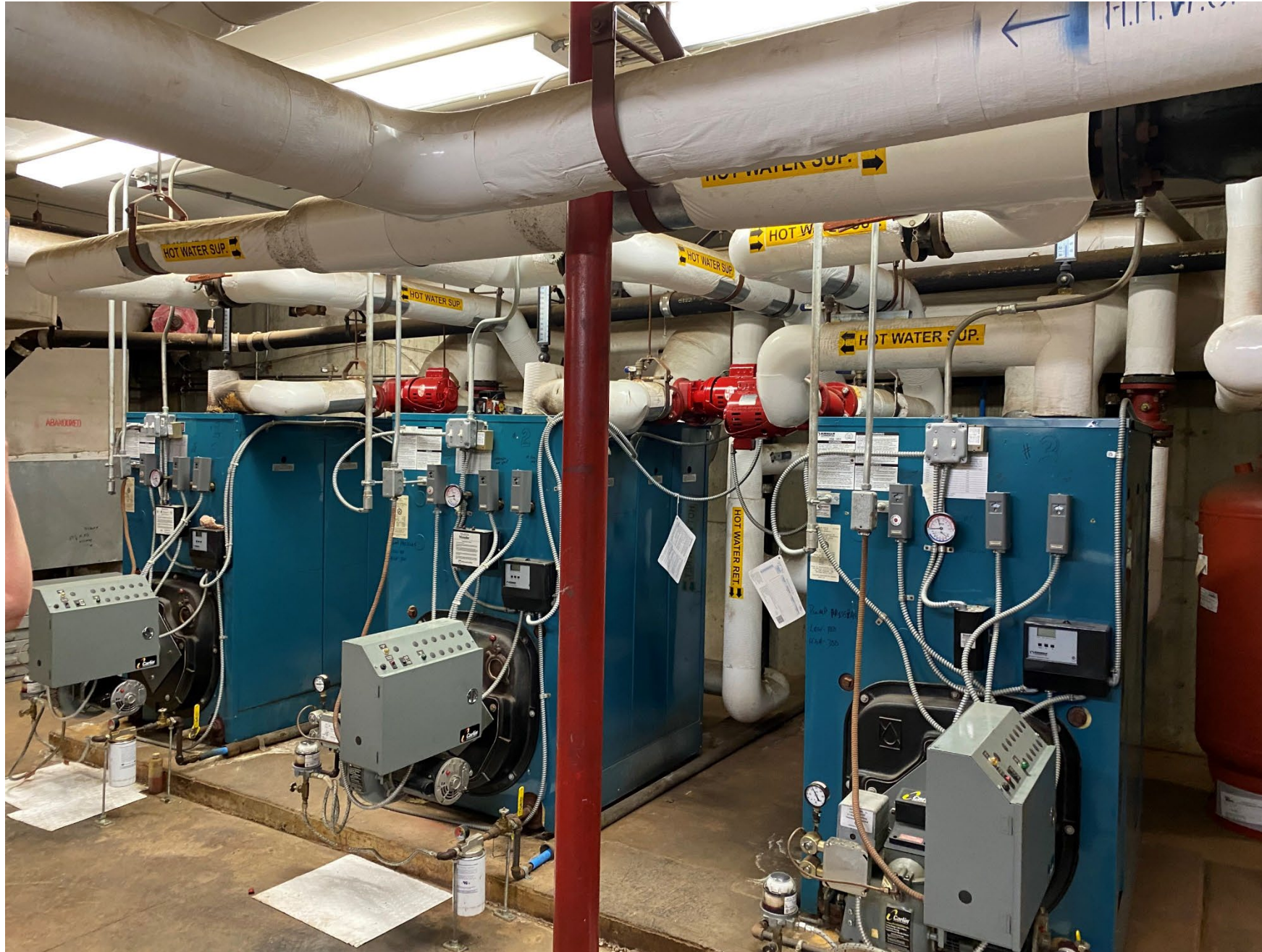
THREE EXISTING BOILERS, ONE NOT WORKING.
