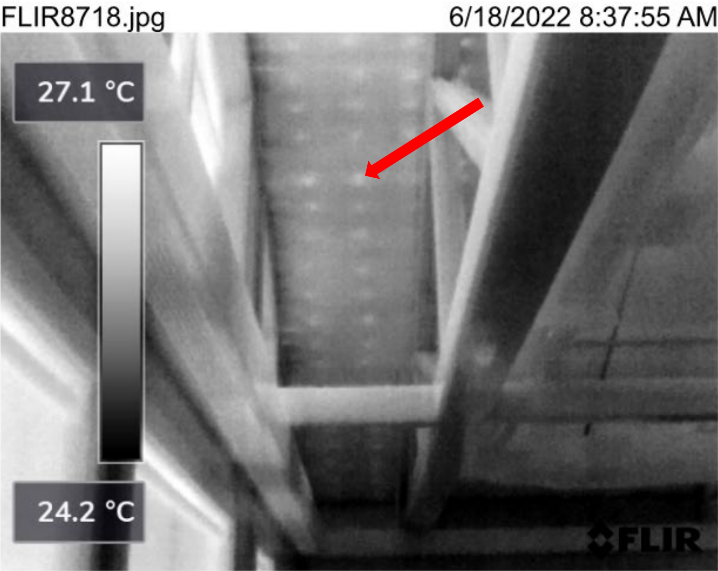
LIKELY AIR LEAKAGE AT ROOFING FASTENERS, VISIBLE IN A REGULAR PATTERN
